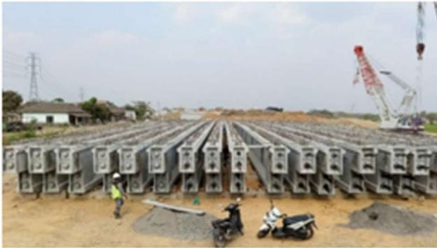
**Gambar 4.** PCI Girder di Stockyard
